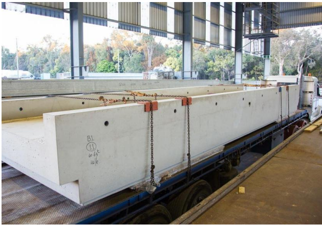
Figure 2 – EFC beams being transported to site and installed.
