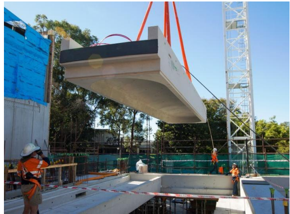
Figure 2 – EFC beams being transported to site and installed.
