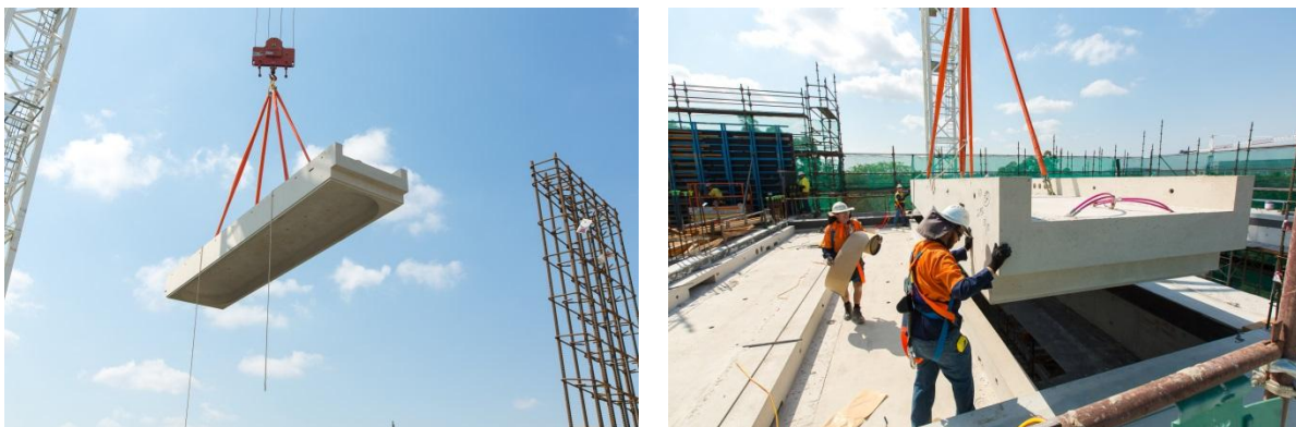
Figure 8 Precast geopolymer beams installation
