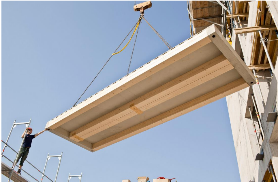
Fig 2. Timber concrete composite floor panel
