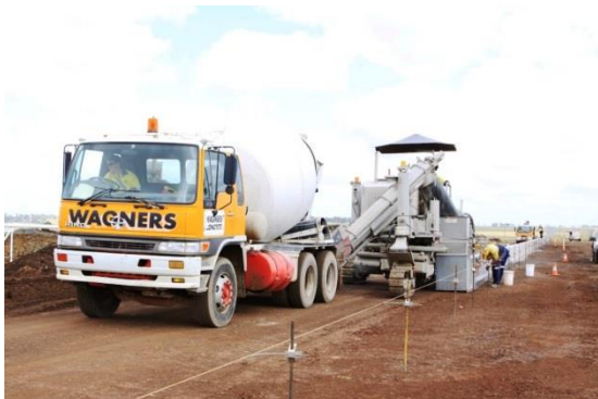
Figure 9. Other Geopolymer Concrete Works at BWWA.
