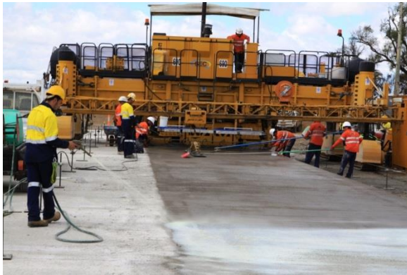
Figure 6. Curing and side forms with dowels.
